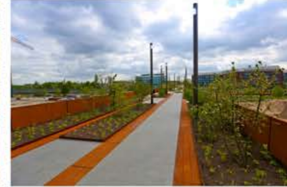
ref. rails kraanbaan
